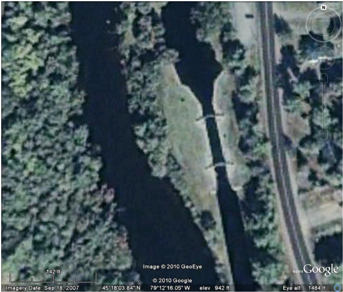
Google Earth aerial view of Huntsville Lock Note that this lock has balance beams on the gates. Rte. 2 is just to the right
