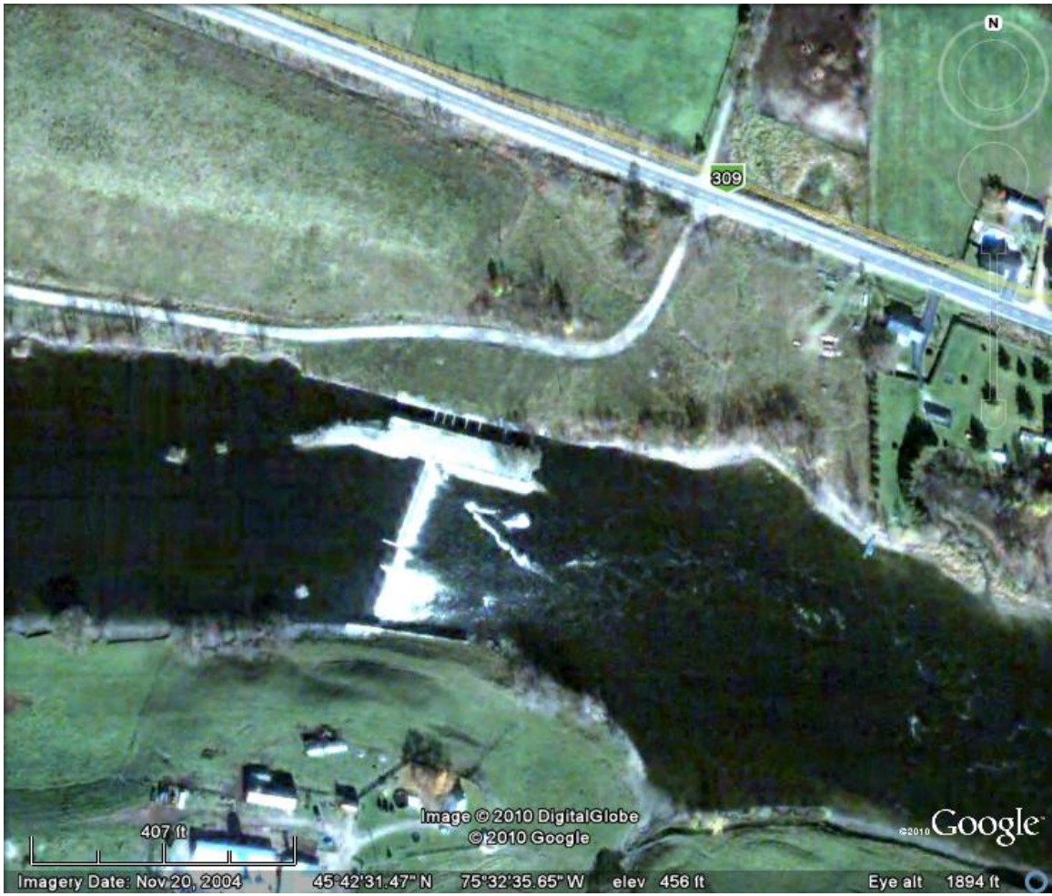
Google Earth view of Poupore, Quebec Dam & Lock
