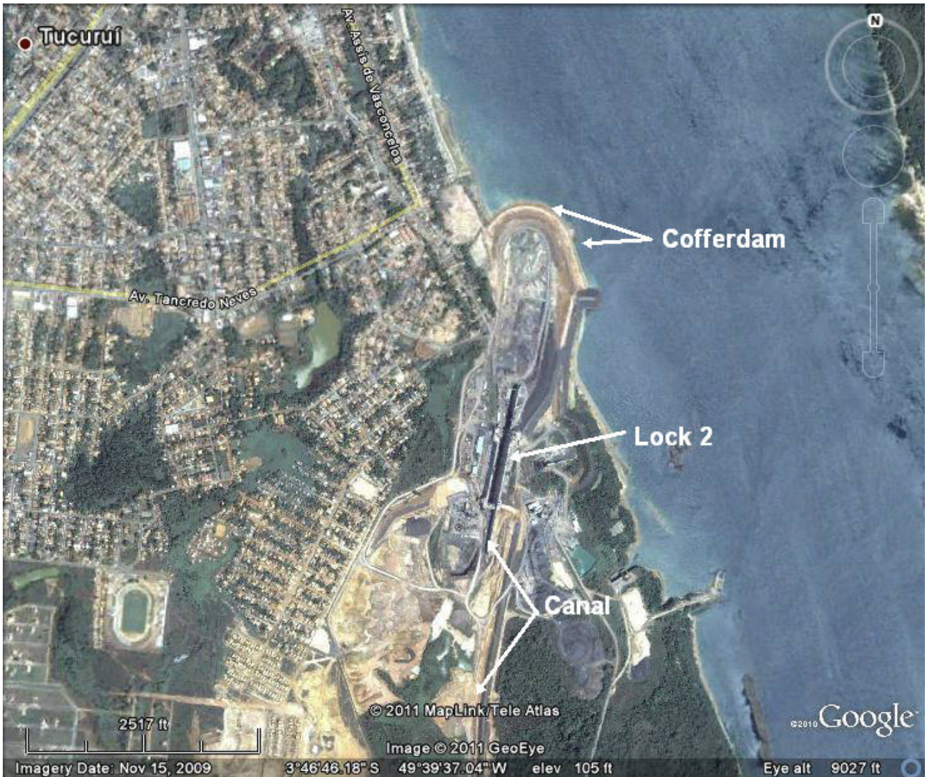
Aerial of Lock 2 at the northern end of the canal
