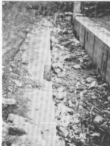
Dismantling process at Lock #2.
