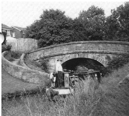
Jeremy Scanlon and his narrow boat on the Macclesfield Canal, preparing to pass under a "Roving Bridge". (In Pennsylvania we would have called this a "Winding Bridge," where the tow-path changes sides of the Canal. WHS)
