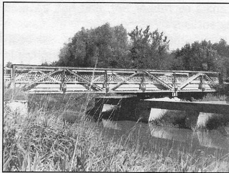
The only remaining swing bridge
