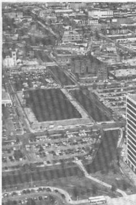
Shown here is the section of the Indiana Central Canal (also known as the Indianapolis Water Company Canal) in downtown Indianapolis, being considered for a canal park.
