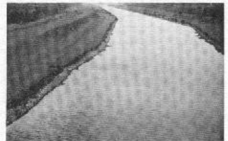
The Cross-Florida Barge Canal, 150' wide, 12' deep, looking east toward Buckman Lock. (Photo taken from Project Bridge SR #19 by Alden Gould.)
