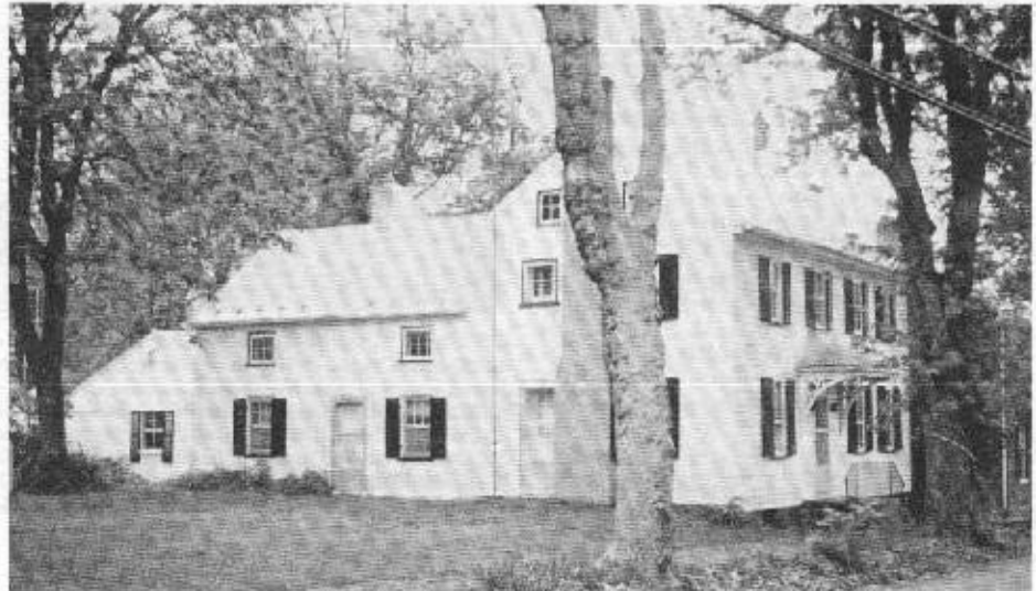
New home of Tom and Nat Hahn in Shepherdstown, West Virginia, a few miles north of historic Harpers Ferry — also new headquarters for the American Canal Society.
