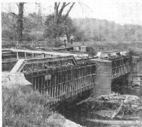
Tinker's Creek Aqueduct
