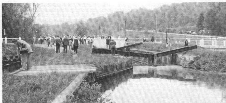
"14-Mile Lock" on the Ohio & Erie Canal at Alexander Mill. (Note one avid canal buff checking the waste-weir at left.)
