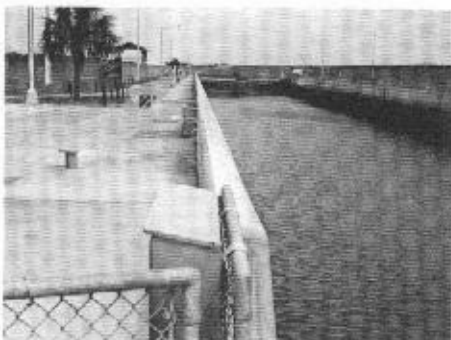
Buckman Lock, 84' x 600', looking east from the west gate. (Photo by Alden Gould.)
