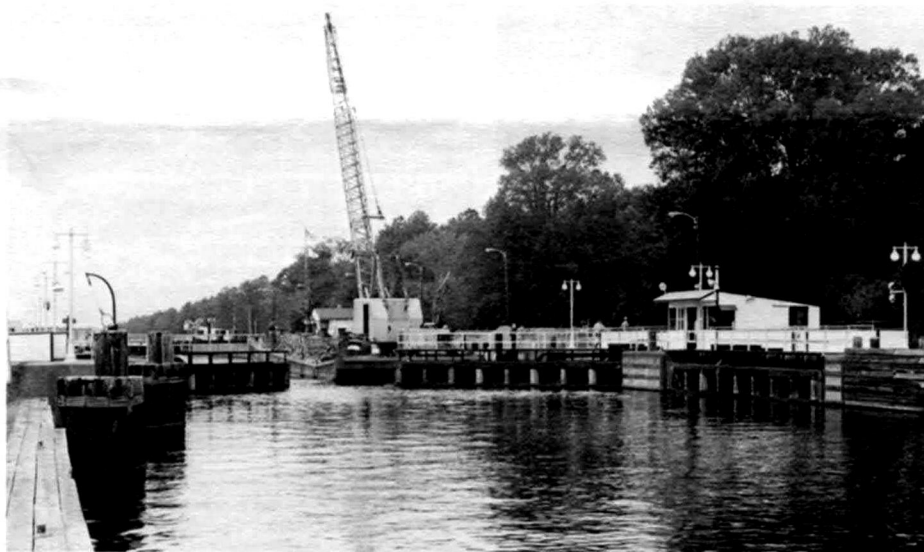
The Albemarle and Chesapeake Canal Guard Lock at Great Bridge, Virginia. Looking west toward the 600-foot chamber. In the foreground is the east end of the lock leading to the Virginia Cut. In the distance can be seen the west end gate opening on the Southern Branch of the Elizabeth River. Note the reversible head double gates in the foreground. The lock is being closed by inside gates, showing the water lighter at that moment in the Elizabeth River. The outside gates are folded back in recesses in the walls. (Photograph, A.C. Brown.)
