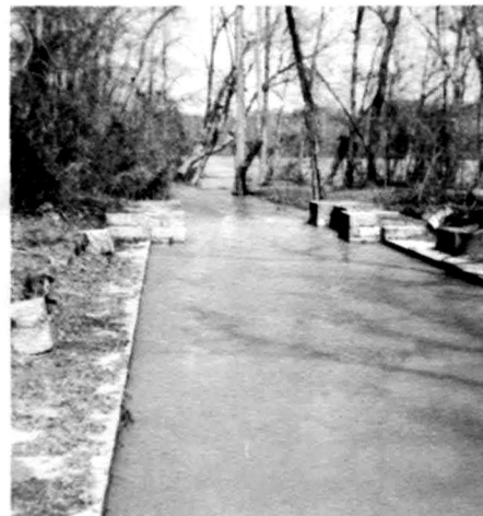
Guard Lock near the dam and river at Landsford Canal, looking north, during a flood 3/22/75 which completely filled the lock. (Photo by Jim Work, Park Superintendent.)
