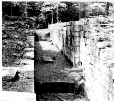
The masonry of Lock Number Two is in excellent condition. In the foreground is the unusual, curved breastwork of Lock Number Three. (Gould photo.)
