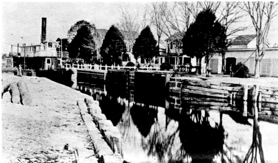
The steamer COMET in the Great Bridge lock in 1895. This rare photograph shows the original gate arrangement and stone work.
