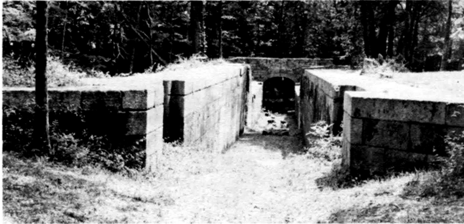
Looking south, with Lock Two in the foreground, Lock Three in the distance, a two-lock combination. Note bridge of lower end of Lock Three. (Gould photo.)
