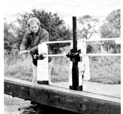
Bob Shopland, Editor, Waterways World , has no trouble with the old mechanical ratchet gate paddle gear of Marsworth Lock 41 on the Grand Union Canal.
