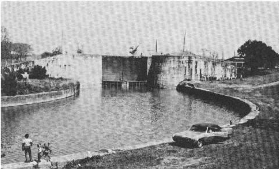
Plaquemine Lock from the Bayou. Note the short pair of gates in front for operating under "reverse head". (W. E. Trout)
