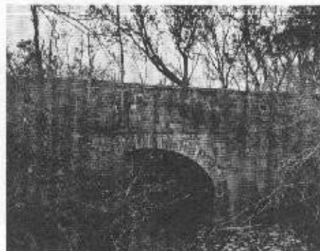
Chockoyotte Creek Aqueduct (Weldon Aqueduct) at Weldon, N.C. (Army Engineer District, Wilmington)
