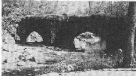
Espada Aqueduct, San Antonio, Texas. (Photo by Bill Trout)
