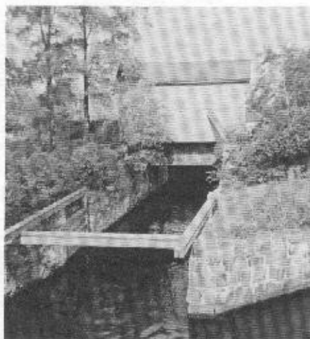
Francis Folly at Lowell, Massachusetts, built in 1848 and reconstructed in 1870 was built to hold back flood waters. Lowered in 1936, it held back a 28 foot wall of water, saving the city of Lowell. (Photo by Aiden Gould)
