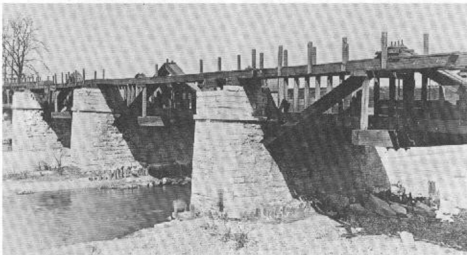
Remains of old aqueduct on the M. & E., crossing the Mad River at Dayton, Ohio. The "King post" support structure is clearly visible. Photo made March 23, 1911.
