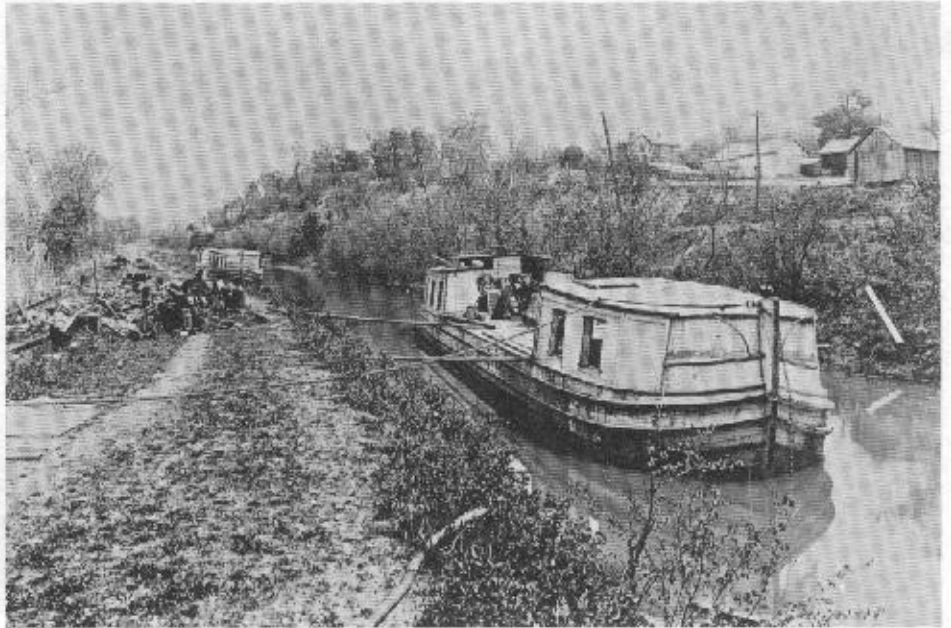
This photo, made north of Miamisburg, looking toward Carrolltown in July of 1904, shows canal freighters reduced to the ignominious task of dumping rubbish along the banks of the canal. Where were the environmentalists, then?
