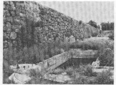
This extant 800' long dam was built by the Tremont Iron Works in 1845 to impound water to power its many iron operations at Wareham, Massachusetts. (Alden Gould)
