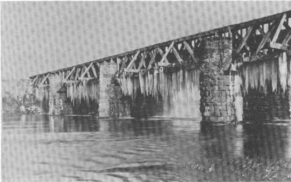
1898 photo of the Walhonding Aqueduct in winter. The icicles are a result of water leakage from the canal flume.
