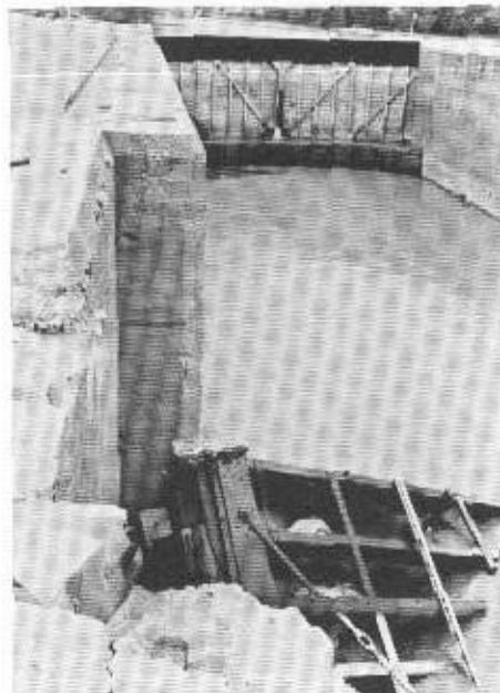
Lock #11, Kentucky River, showing gate washed off, May 1977. (Photo by Bill Trout.)
