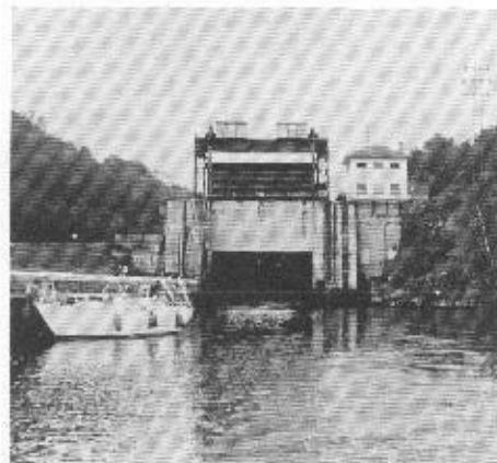
A guillotine-type lock on the Erie Barge Canal near Little Falls, N.Y. The upper gate is the conventional mitre-type, but the lift of the lock is so great, nearly 45 feet, that the lower gate raises up like an elevator, high enough to allow the superstructures of the boats to pass under it. Passengers on deck enjoy an unexpected shower-bath!
