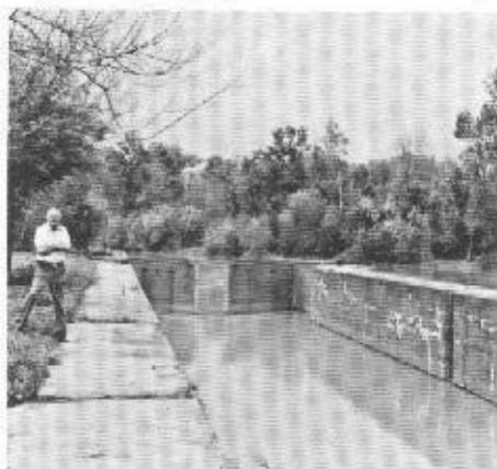
William McClellan on the first concrete river lock on Rough River , a branch of the Green , in Kentucky. (Photo by Bill Trout.)
