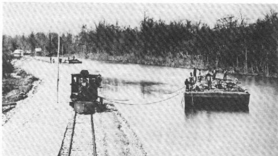
Work barge and repair crew, under tow on the Muscle Shoals Canal, February, 1892. (Photo courtesy, David Wilson, Jackson, Tenn.)
