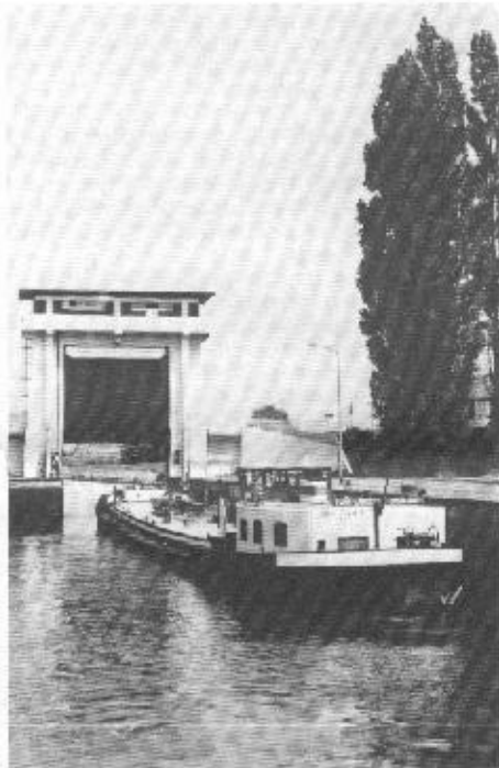
Gullotline lock on the South Williams Canal, electrical and modern.
