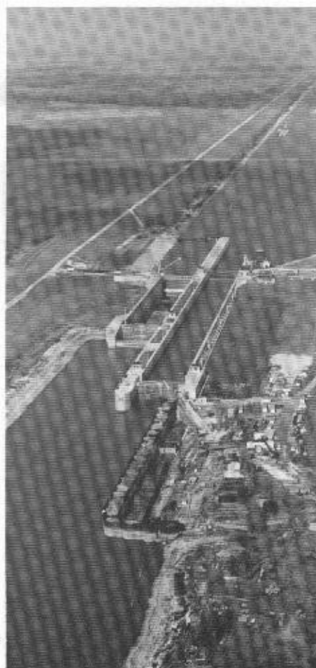
This unusual photograph is of Locks 27 (mile 185.1) of the Chain of Rocks Canal (mile 184.2-194.0) of the Mississippi River. The locks are near Granite City, Illinois. (Submitted by John Purcey of "Scientific American.")
