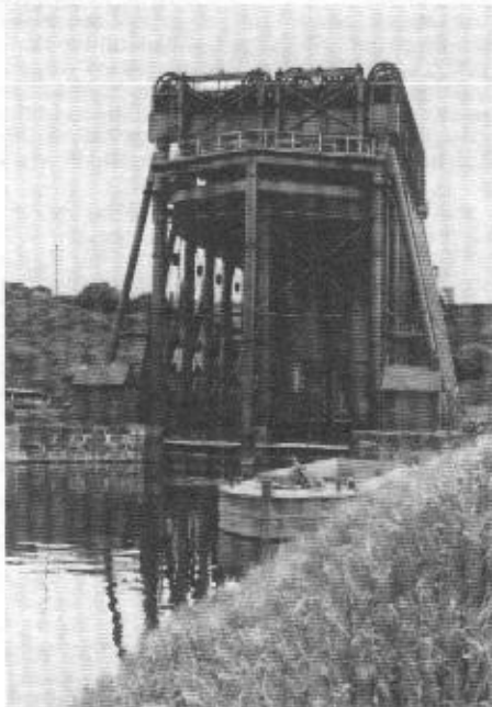
One of England's outstanding canal engineering structures is the Anderson Lift in Cheshire built by Leader Williams in 1875 to connect the Trent & Mersey Canal with the Weaver Navigation 50 feet below.
