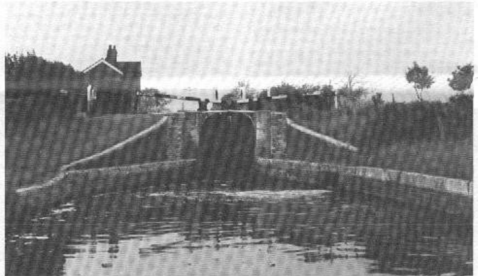
A typical English canal lock (Aston Lock) from below on the Trent & Mersey Canal in Staffordshire. Note the brick lockhouse to the left, the handy stairs on each side of the lock, and the rise for the tow animal on the left.
