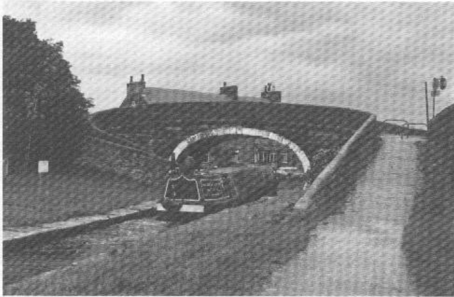
Nothing is more beautiful than the graceful English canal bridges. This changeover bridge (Bridge No. 1) near Marple, Cheshire on the Macclesfield Canal permits the changing of the towpath from one side to another.
