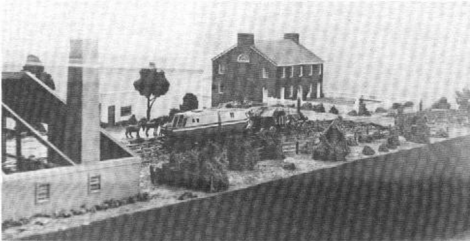
Part of the new model of Plane Number Six, built by Fred Connacher. The steam-driven engine house, at the head of Plane Six, is shown at the left. A sectional canal boat train is shown, being hitched to one of the APRR steam locomotives, for the horizontal Allegheny Summit run. Lemon House is shown in the background.
