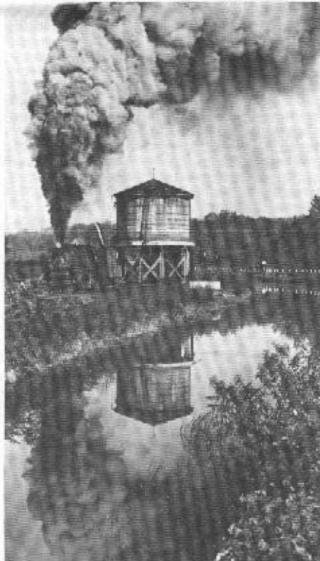
This photo from "Champlain to Chesapeake" illustrates the side-by-side competition of canals and railroads, along one of the Delaware Canals in the Lambertville-New Hope area. McKelvey identifies the location as "near Jacob Creek Road".
