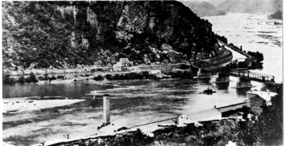
This 100-year old photo taken from Harpers Ferry shows the C. & O. Canal on the northeast bank of the Potomac River. In the center of the photo is lockhouse for Lock 33, and behind it the old Salty Dog Saloon. At the right is the famous old Bollman truss bridge, erected in 1852 as part of the B. & O. railroad system. (Courtesy of John C. Frye, Gapland, Maryland.)
