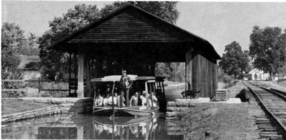
The rejuvenated Whitewater Canal Aqueduct at Metamora, Indiana, thought to be the only covered-bridge type wooden canal aqueduct still in existence anywhere in the world. The "Valley Bell" canal boat shown here carries about 35 passengers along a fully watered section of the "Whitewater" and through a lock at the edge of town. (Photo courtesy of Eugene R. Bock.)
