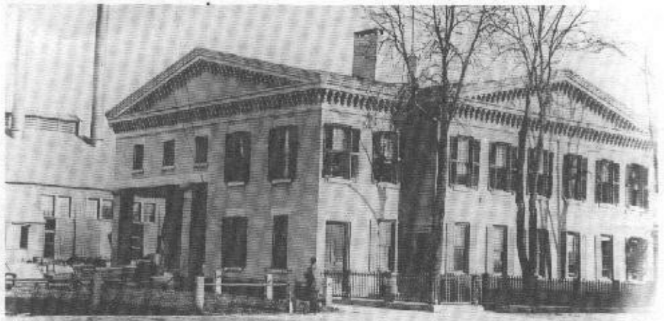
The Weigh-Lock building on the Erie Canal at Syracuse, New York in the late 1890's. A canal boat can be seen at the left, entering the weigh-lock, at the rear of the building. The canal is gone, but the building is now the headquarters for Canal Museum Associates, used primarily for canal displays and exhibits. The new administration annex is located out of the picture to the right.
