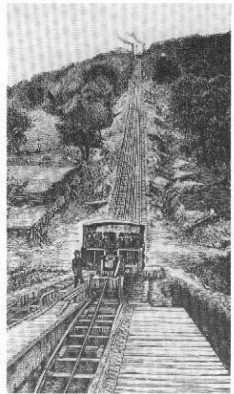
This old print of the Mount Pisgah Inclined Plane on the famous "Switch-Back" Railroad, serving the Lehigh Canal at Mauch Chunk, typifies the many inclined planes in use on the primitive railroads in Pennsylvania before the advent of the steam locomotive.
