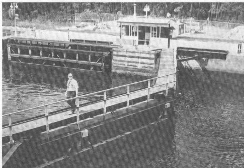
Detail of the west end gates of the Albemarle and Chesapeake Canal lock at Great Bridge, Virginia in 1973. It appears that it was low tide in the Southern Branch of the Elizabeth River, and high water in the lock and the Virginia Cut of the A&C Canal. (Photo by Alexander C. Brown)
