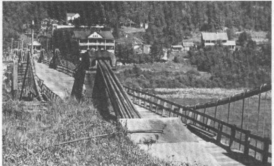
John Roebling's 1848 Aqueduct, on the Delaware and Hudson Canal, was converted into a highway bridge when the canal was abandoned.
