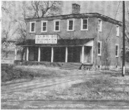
Front view of the Lockhouse in Havre de Grace, now being restored and re-furnished. (Photos by Bill Shank)
