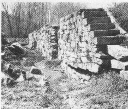
Ruins of Locks Number 46 and 47 below Lynchburg, at the Rope Ferry. Locks were rubble stone, lined with planking, built in 1840. (John Taylor photo).
