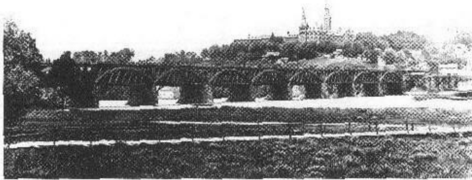
Potomac Aqueduct of the Alexandria Canal sometime after 1867, when a highway toll bridge had been constructed above the canal trough, making it a two-tier structure. View from the Virginia side of the river, with the Georgetown University campus in the background. (Library of Congress photo.)
