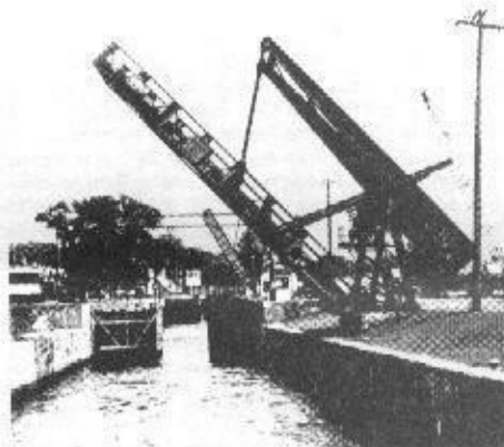
An array of draw-bridges greeted us at Lock #1 on the Oswego canal at Phoenix, N.Y. View into the lock chamber as we departed, downstream. Lock Lift: 10.2 ft.
