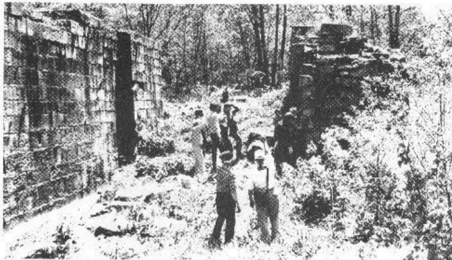
Virginia Canals and Navigations Tour Group inspects Blue Ridge Dam and Guard Lock on the J. R. and K. near Glasgow, Virginia. (Photo by Bill Shank)
