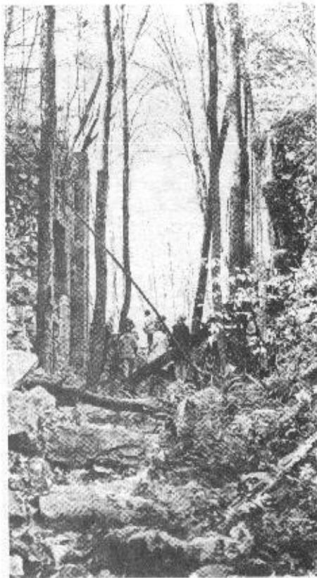
Lock No. 6 on the Feeder, highest lock on the entire Union Canal system. This lock will be torn down by the park contractors, due to hazard of falling masonry.
