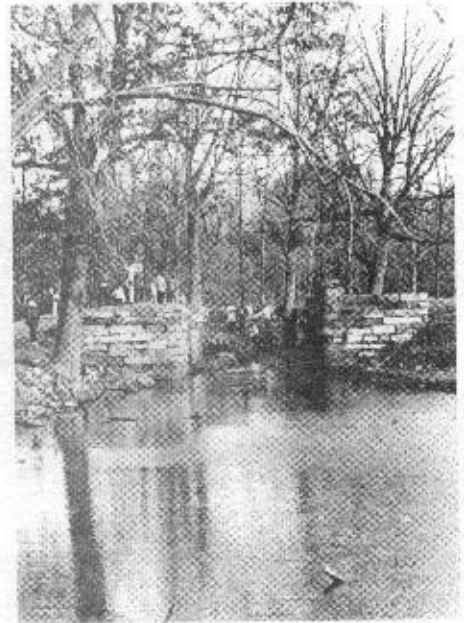
Lock No. 21 West on the Union Canal, during the visit of the PCS-CSNJ buses. Directly behind this lock are ruins of the Swatara Creek Aqueduct.
