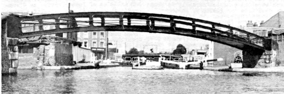
Under this unusual pedestrian bridge can be seen a pair of operating locks on the Regent's Canal in the Camden-Town section of northern London. Bill Shank snapped this photo from one of Jason's Narrow Boats while touring southern England this past June. The balance-beam lock gates shown here are almost identical to those in use on American canals a century ago.
