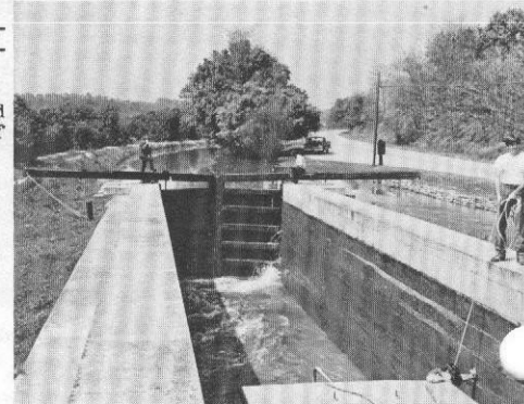
Fully restored lock on the "Whitewater" at Metamora, Indiana. The "Valley Bell" tour boat (lower right) is being locked through. (Eugene R. Bock photo.)
