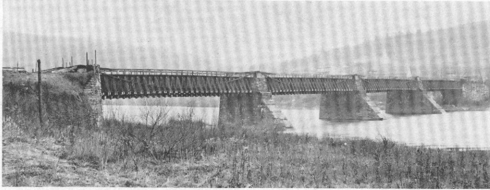
The Roebling Aqueduct across the Delaware River, from the New York State side, circa 1900, shortly after the Delaware and Hudson Canal had been abandoned. The old structure, still standing today, has been converted into a toll bridge.
