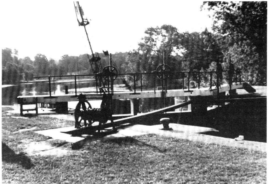
Hand-operated, lower-gate mechanism of the flight of locks on the Rideau at Jones Falls, Ontario. (Photo by Bill Shank).
