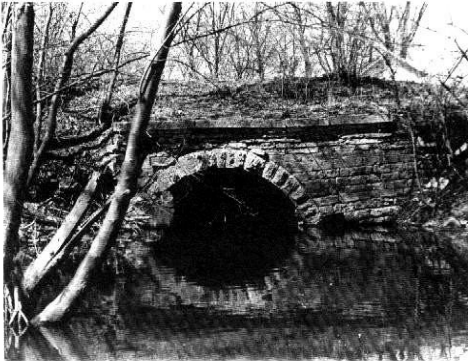
Tom and Julia Meek, active promoters of the new Indiana Canal Society, have for the past several years been exploring various sections of the Wabash and Erie Canal in Indiana. Here is one of their photos of the well-preserved "Culvert Number 73" where the W and E crosses Prairie Creek (formerly La Fontaine's Creek) near Onward, Indiana.
