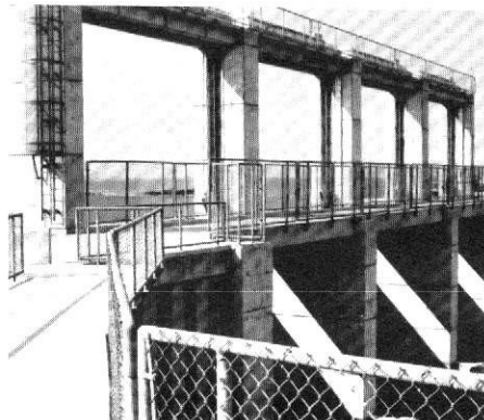
Detailed view of the manually-operated sector gates of the Port Mayaca Lock. Lake Okeechobee can be seen in the background.
