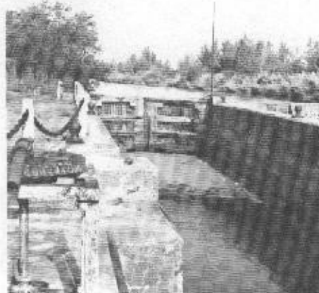
Lock Number One on the North New River Canal, Fort Lauderdale, Florida which operated as part of the Everglades Drainage District 1912-1930. The old lock (130' x 25') is in excellent condition.
