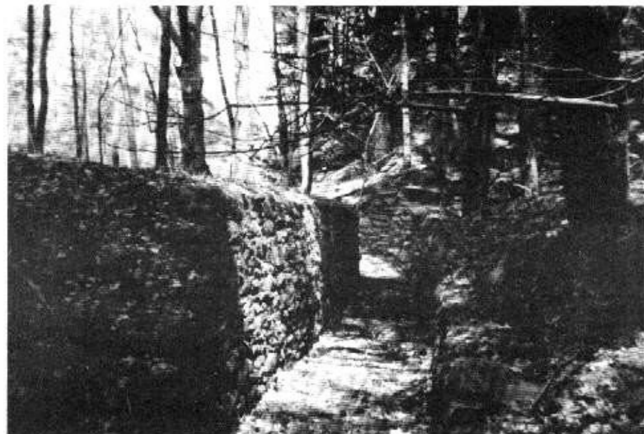
Joe Brolley, of Wilkes-Barre, Pa., has once again provided us with an interesting canal photo from his area. Pictured here is his photo of the well-preserved waste weir near Lock #23 on the Delaware and Hudson Canal at Kimble, along the Lackawaxen River, Wayne County, Pa.
