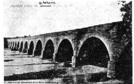
An old print of the Schoharie Creek Aqueduct of the Erie Canal at Fort Hunter, N. Y., built in 1841 of cut limestone -- 624 feet in length.
