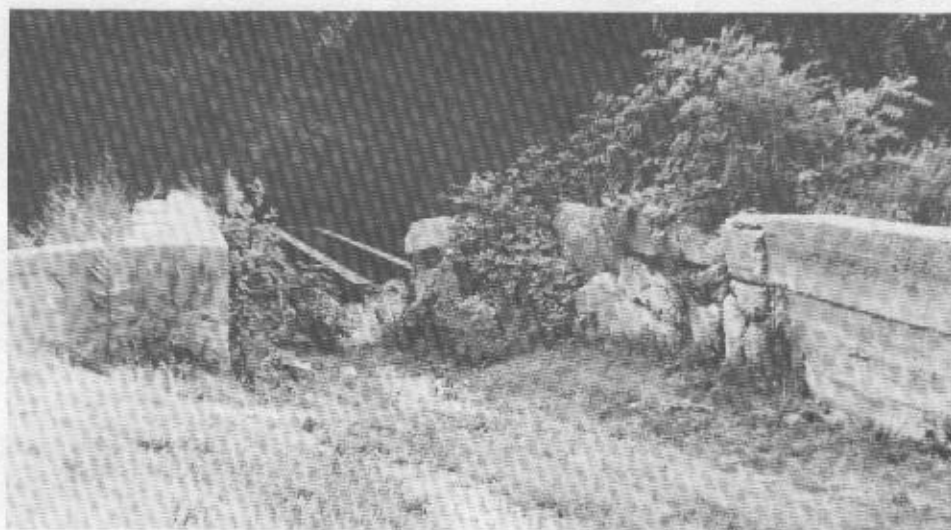
Ruins of the Clinton-Kalamazoo Canal, Yates Cider Mill, Rochester, June 1982. In the background are several metal beams which helped support the old Aqueduct over the Clinton River just below. (Photo by Howland Fisk.)
