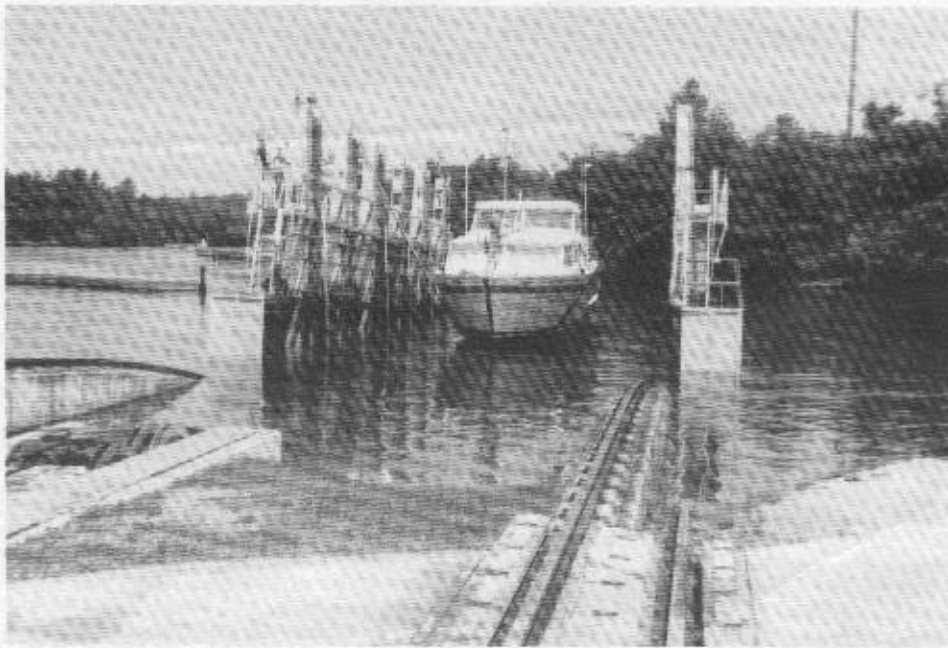
Boat Carriage at Big Chute showing the double tracks entering the water beneath it.
