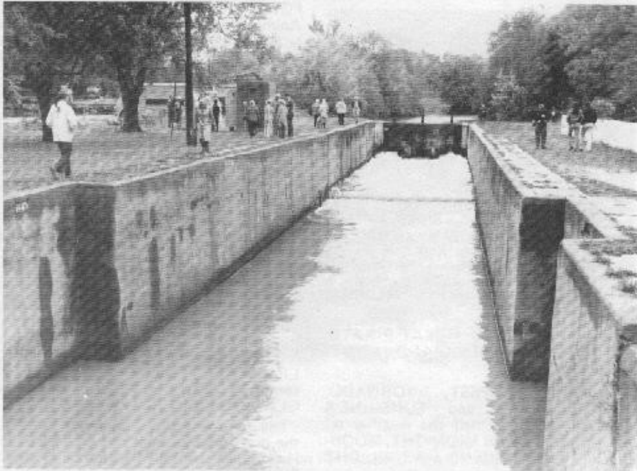
Typical cement-lined lock on the Delaware and Raritan Canal as it appears today. The upper gate has been replaced by a weir, with wicket gates to control the flow of water. (Photo by Bill Shank)
