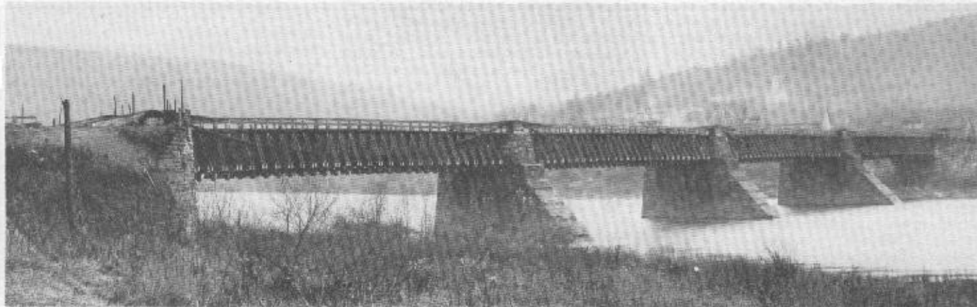
The Roebling Aqueduct on the Delaware and Hudson Canal (Circa 1898) when it still carried water across the Delaware River at Lackawaxen, Pa. The water flume has since been removed, and the structure has been used as a highway toll bridge for eighty years.
