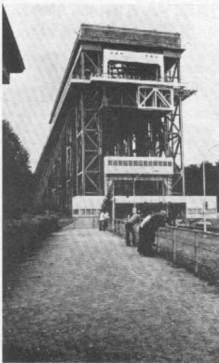
The Neiderfinow Lift presents an imposing appearance from the lower level. It has a lift of 116 feet, handling 1000-ton vessels.
