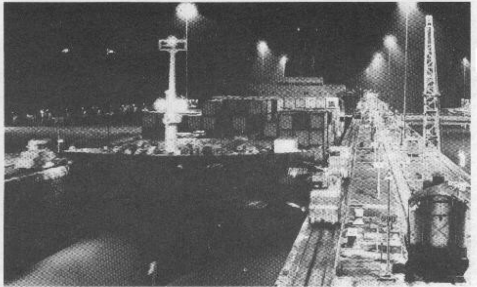
Newly installed, high-mast, high-intensity lighting at Miraflores Locks extends the hours during which large vessels can pass through.
