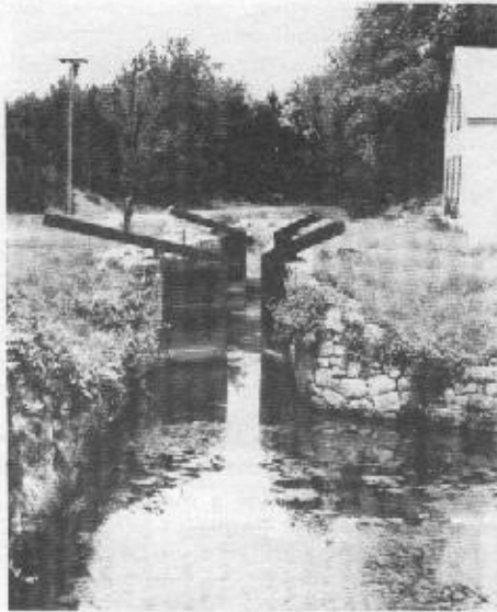
Lock Twelve on the Farmington Canal at Cheshire, Connecticut as rebuilt in 1977. Locktender's house on the right. To view this site, take Route 44 off Route 10 from Cheshire to Railroad crossing. Lock is about 500 feet left of RR crossing. (Photo by George Wills, Lebanon, Pa.)
