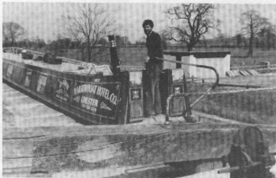
Mike Hobbs at the tiller, while passing through one of the narrow, single-gate locks. Note wicket-gate hardware in the right foreground.
