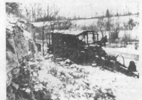
Some of the steam shovels were brought north after the Panama Canal was finished. This one was finally abandoned after long years of service in a Canadian stone quarry.
