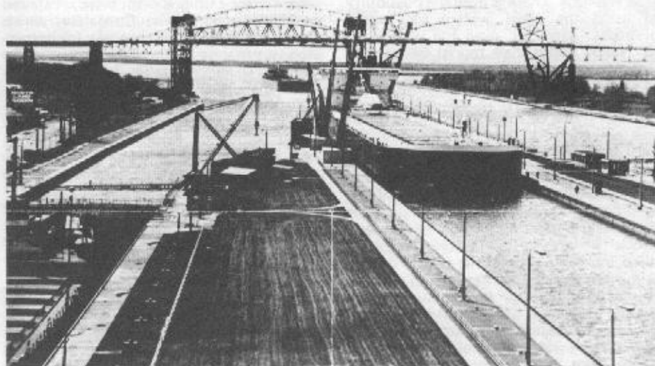
Our Great Lakes photographer, Bill Etchberger, has just returned from another trip to Saulte Ste. Marie where he obtained this interesting picture. Taken from between Poe and McArthur Locks, looking west, it shows an extremely large freighter nudging its way into Poe Lock, with mere inches to spare on both sides. The two other American Locks - Davis and Sabin - are out of the photo to the right.
