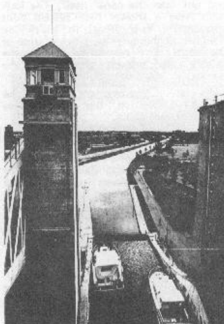
A view looking downstream from the upper deck of the famous Peterborough Hydraulic Lift Locks. Several small boats are shown being lowered 65 feet from one canal level to the other.
