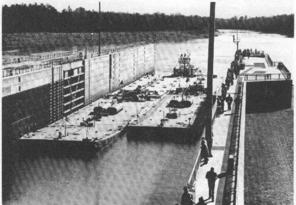
Scene at the Columbus, Mississippi Lock and Dam on the Tenn-Tom, January 18, 1985. The "Tow" of the Waxler Towing Company of Memphis is shown edging its way into the 110-foot wide by 600-foot long lock, which is standard for all ten locks on the Tenn-Tom.
