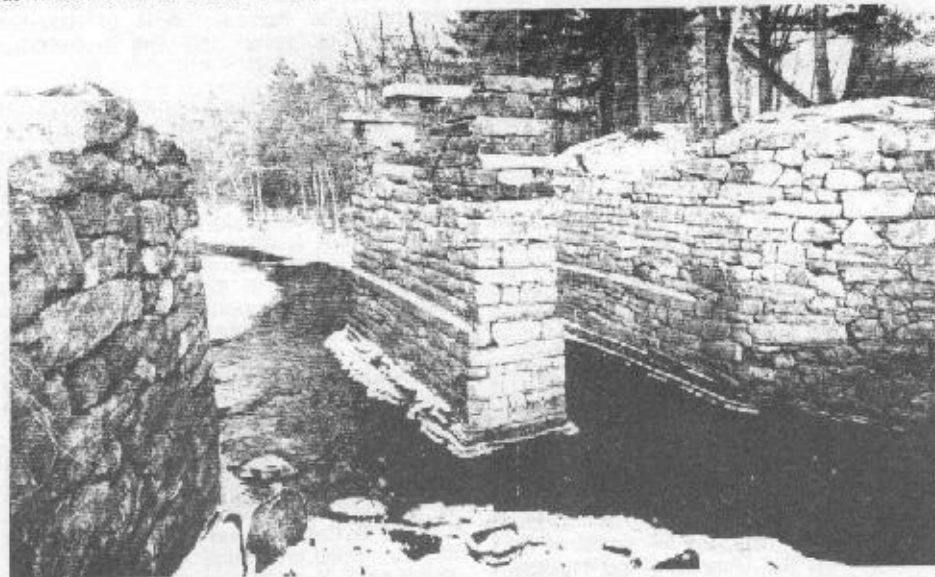
Ruins of the Middlesex Canal Aqueduct, which carried canal boats over the Shawsheen River. The site has been declared a National Historic Civil Engineering Landmark, and stabilization work has been done here.
