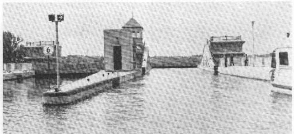
Looking back from the stern of our tour boat as we leave the Peterborough Lift Lock at the upper level of the canal. No complex mechanism is needed to activate the lift - merely an extra foot of water in whichever of the two chambers is in the "up" position; the extra water weight activates the lift.
