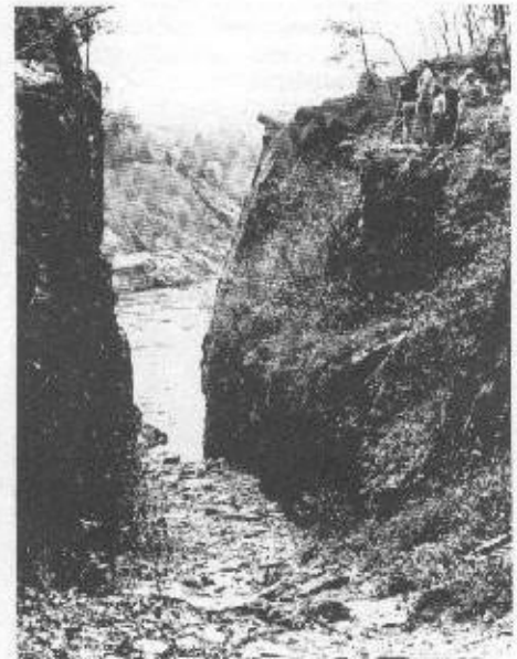
The final tremendous "cut" through solid rock to get the canal back to the river below the falls. With the crude blasting equipment of the late 1700's this must have been a heart-breaking task!
