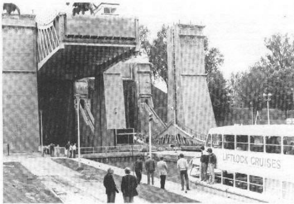
Our tour boat ties up while our party inspects the World's Highest Hydraulic Lift Lock. Minutes after this picture was made our boat entered the 33-foot wide by 140-foot long chamber shown in raised position on the left.
