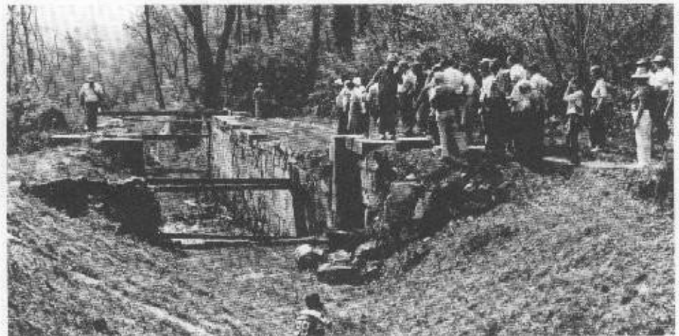
Here is one of the stabilized locks at the lower end of the Great Falls Canal. This is one of the five locks which lowered the boats to the Potomac River downstream from Great Falls. Average drop in the locks was about 16 feet per lock, a total of 77 feet.
