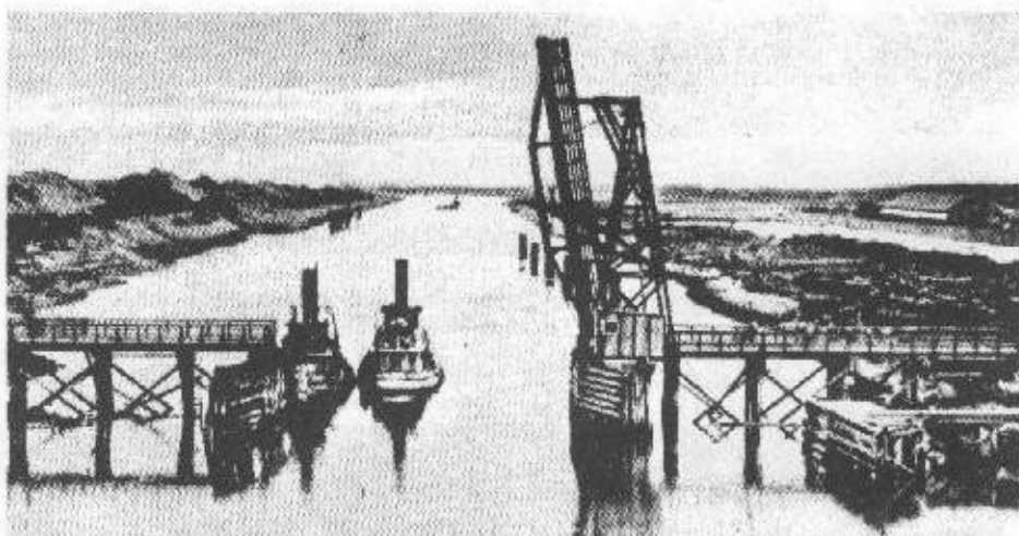
Completed section of the 17-mile long canal connecting Buzzards Bay and Cape Cod Bay, near the Cape Cod Bay entrance, as it appeared in 1913. A highway drawbridge is prominent in the foreground.
