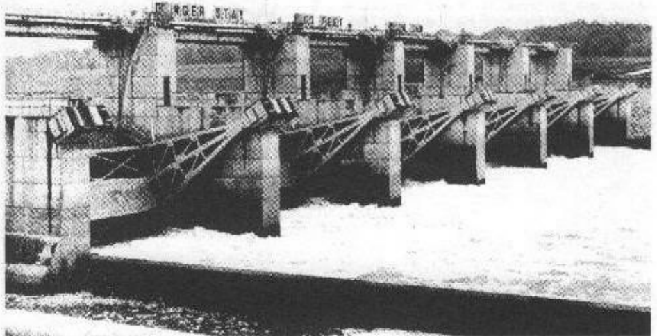
The Aberdeen, Mississippi Dam, which raises the Tenn-Tom Waterway 27 feet, is being considered for a local source of hydro-electric power.
