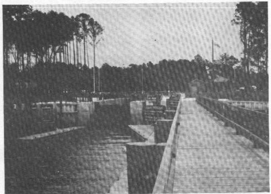
Similar Lock at Windmill Harbour, Hilton Head. View of the lock from the river entrance pier. The lock is reversible for high and low tides.
