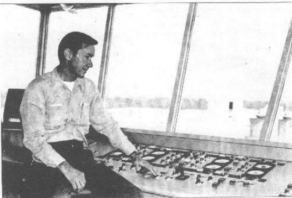
Aberdeen Lock Superintendent Wilson Bobo operates the controls inside the Lockhouse to open and close the gates and valves of the 110-foot wide by 600-foot long lock. (Photo by Rachel Eide.)
