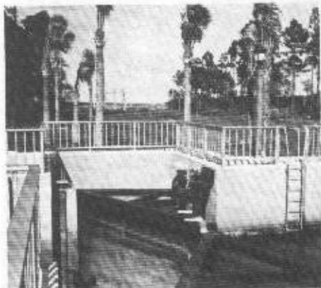
These are the sector gates of the Waxford and Windmill Locks, which operate in either direction, depending upon the tides. (All photos by Dave Barber.)
