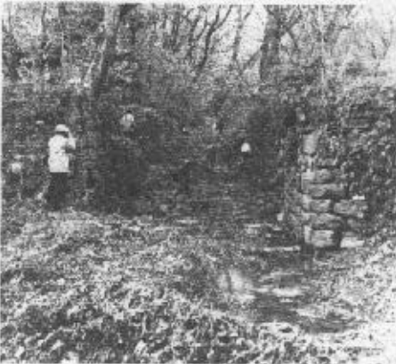
A PCS Group inspects Lock Two ruins on the Conestoga Navigation. Most of the Conestoga was slack-water navigation; there was a dam near this lock.
