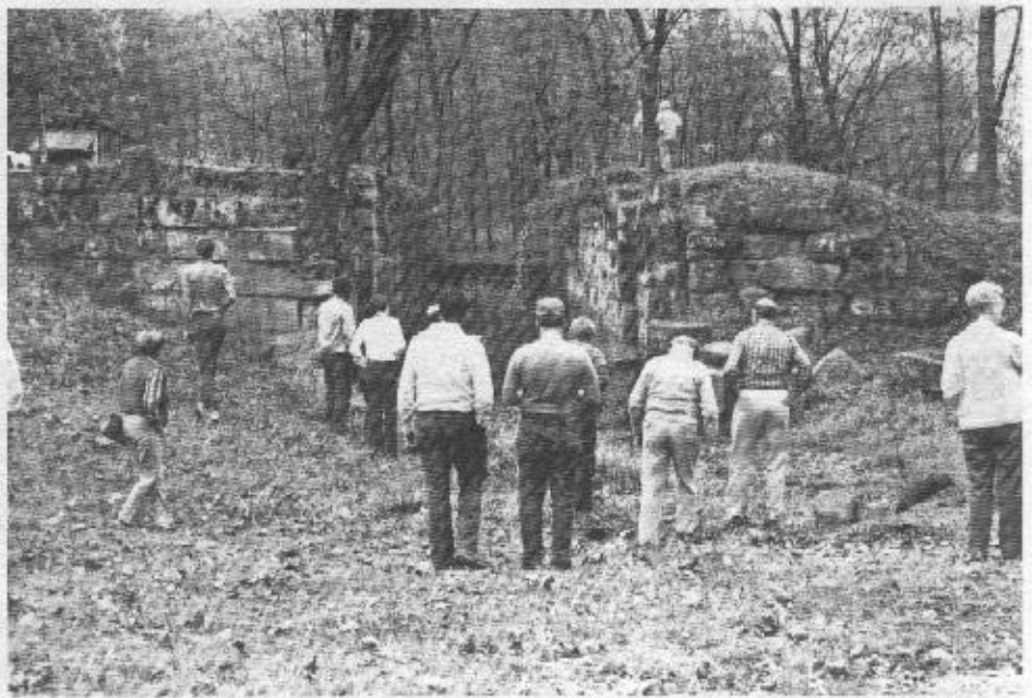
A group of CSO members inspect one of the well-preserved locks of the Hocking Canal, south of Lancaster, Ohio.
