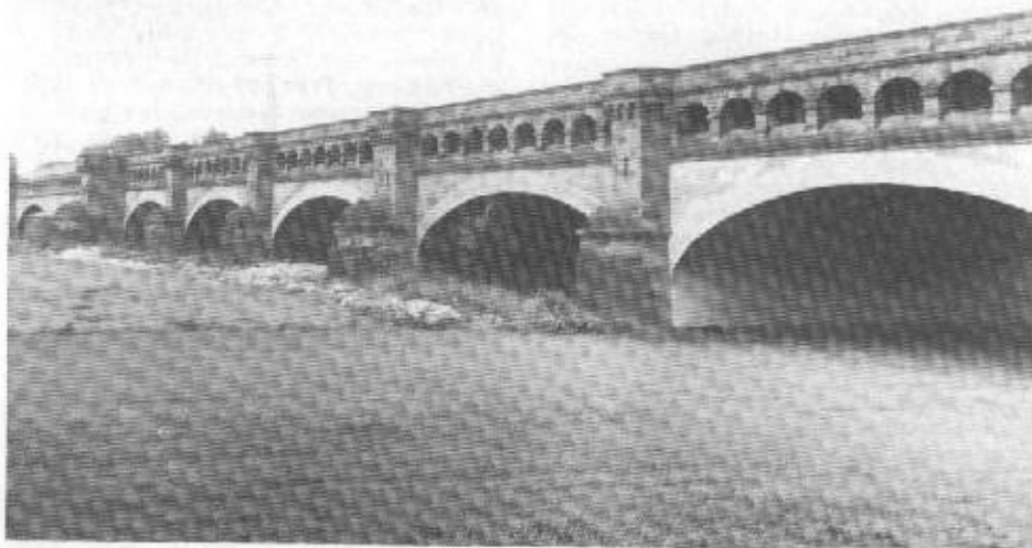
This view of the north side of the Aqueduct shows the difference between the original stone and the modern concrete structure. Since the Minden Aqueduct was built in the age of steam power there was never a need for a tow path. (Photo by Bruce Russell.)
