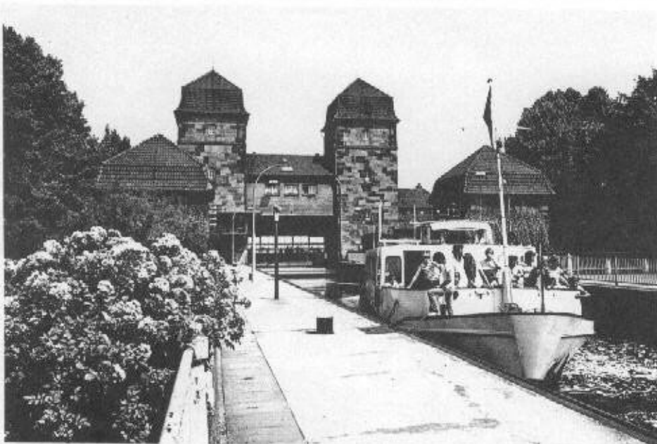
Ornate edifice housing the lift-gate on the Minden Lock, which lowers or raises the boats seventy feet between canal and river levels. The lock is shown full, in this view, lift gate closed.
