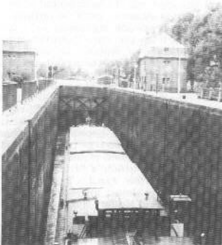
View of a Polish boat in the main lock chamber at Minden. It is rising from the level of the River Weser to the level of the Mittelland Canal. About 50% of the boats passing through Minden are Polish vessels. The Minden complex also contains a smaller lock used only by pleasure craft. (Photo by Bruce Russell.)
