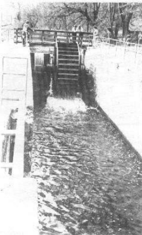
After the canal above Metamora was abandoned for transportation, an over-shot water-wheel was installed in the upper lock to power the old gristmill. Surplus water flows around the Lock, as shown in another photo.
