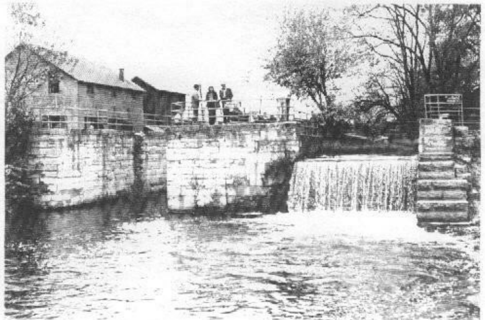
The Metamora Lock and "by-pass" weir shows an adequate supply of water for the canal downstream. In the left background is the old grist mill, powered by canal water.
