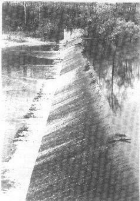
The Laurel Dam rebuilt across the Whitewater River in 1953 to restore water to a ten-mile section of the old canal between Laurel and Metamora, Indiana.
