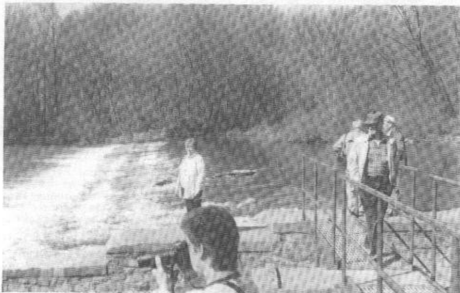
The tour group inspects the Bald Eagle Dam, which feeds water into the Cross-Cut Canal, still maintained by Lock Haven paper plants as a water supply. In the foreground is the re-pointed masonry of the old Log Schute, to by-pass the dam.
