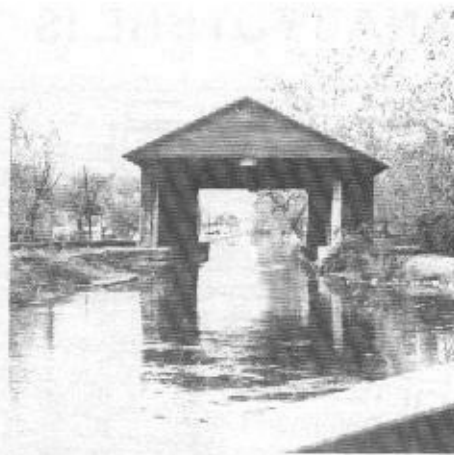
The Duck Creek Aqueduct near Metamora, as seen from the bow of the "Ben Franklin". This is probably the only covered-bridge type aqueduct in the world — still in use.
