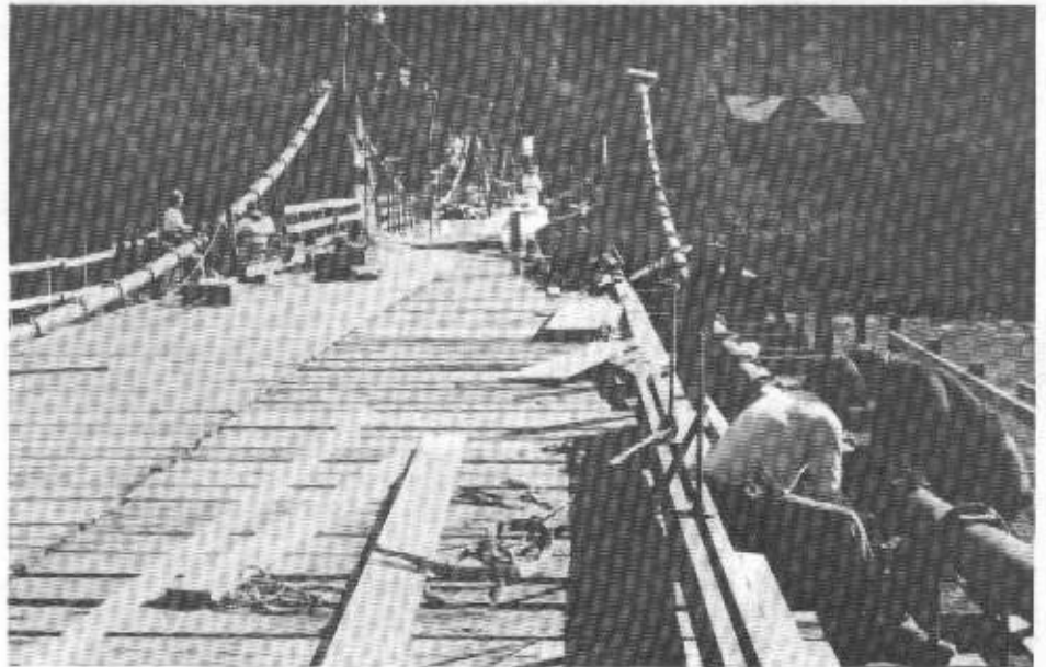
General view of the rebuilding of the old bridge floor.
