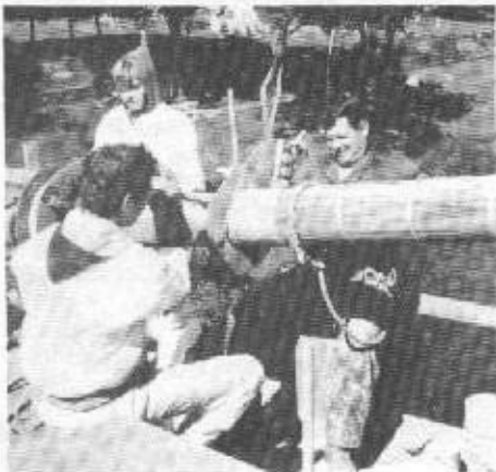
Re-wrapping the old bundled wires with new, galvanized steel wire, a laborious process.
