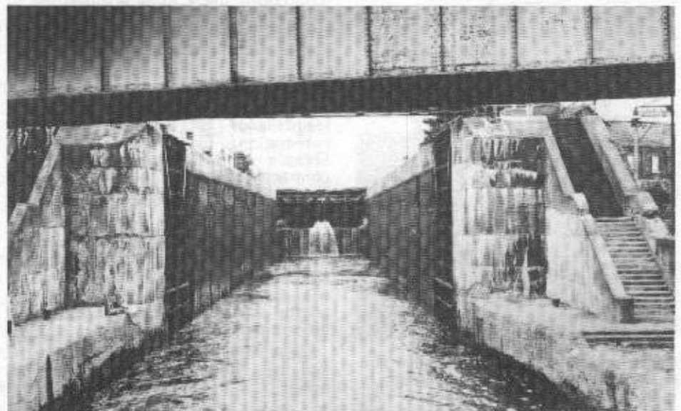
Lock Number Three on the Oswego Canal at Fulton, with a lift of 27 feet.
