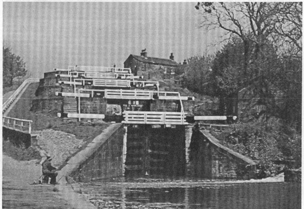
One of the great sights of Britain's waterways -- the Bingley Five-Rise Staircase of Locks, which lifts the Leeds and Liverpool Canal toward its Pennine summit. (Photo by Derek Pratt, courtesy of the British Waterways Board.)
