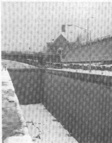
Interior of the upper lock chamber at Lockport, drained for winter maintenance. Note the drains at the bottom of the chamber. (Bruce Russell photo)
