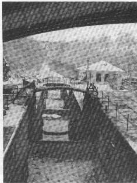
One of the old flight of locks has been preserved as a spillway at Lockport. Miter gates were removed in the 1920's. The control house for the newer gates is at the lower right. (Bruce Russell photo)
