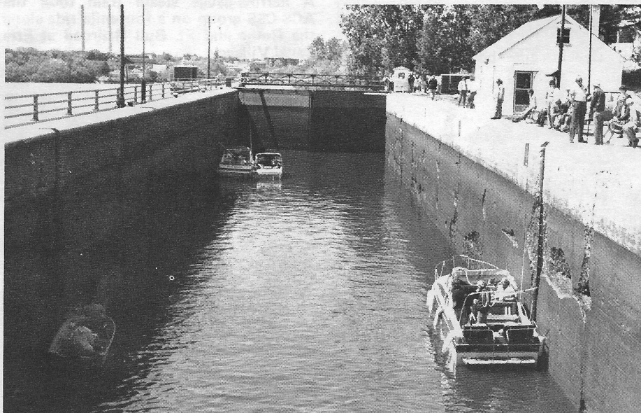
Several small boats bound downstream in one of the high-lift locks on the south outskirts of Oswego.
