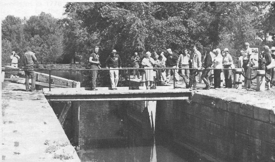
We inspect "Mud-Lock", a well-preserved relic of the Old Oswego Canal, on the north outskirts of Syracuse. Keith Kroon, ACS Tour Chairman, left center of the bridge.
