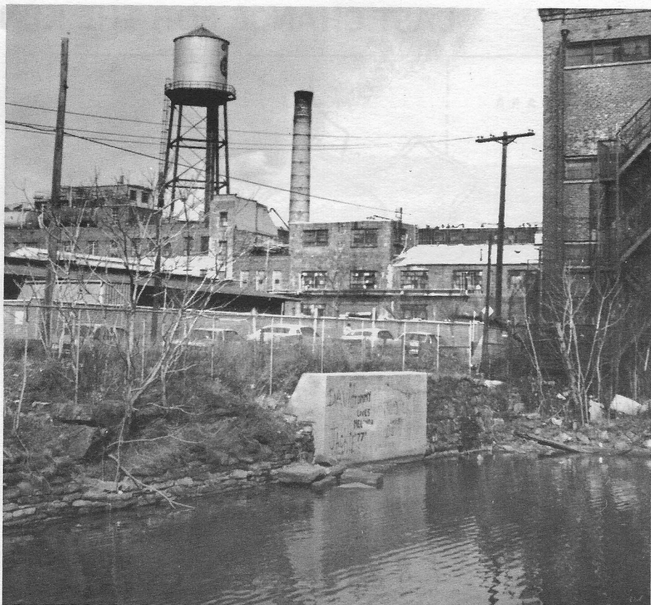
On the extreme western end of the Morris Canal Basin can be seen remnants of a sandstone wall, no doubt going back to the 1840s. The concrete barrier was erected sometime after 1924 when the canal west of the basin was filled in. Nevertheless it denotes the exact spot where the 100 mile waterway officially began. (Russell photo)
