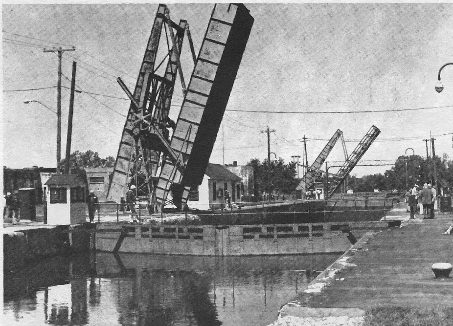
Lock Number One on the presently-operating Oswego Canal presents an array of draw-bridges to the water-traveler.
