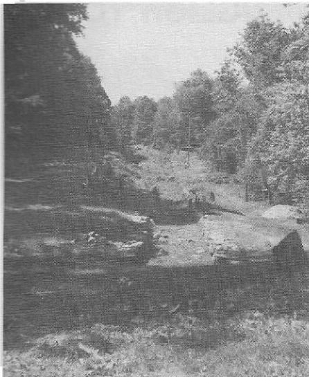
At Ledgewood, one of the Morris Canal's quarter-mile inclined planes is still in excellent state of preservation. The spillway which carried excess water from upper to lower levels is quite apparent to the right of this photo. The bed of the inclined plane is to the left. (Bruce Russell photo.)
