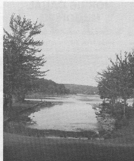
The point at which the Morris Canal boats entered Lake Musconetcong. In the foreground is the small basin which stood at the foot of one of the inclined planes. In the distance, segments of the old tow-path causeway across the Lake are visible. On this causeway, the mules towed the boats across the Lake. (Bruce Russell photo.)
