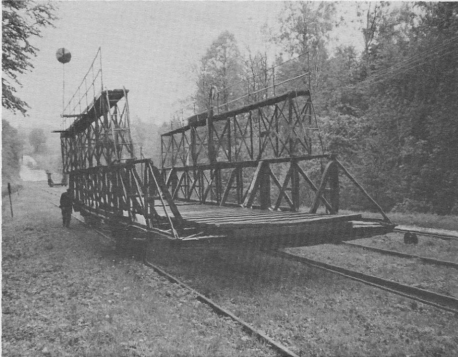
The Buczyniec Incline, with empty boat-carriage in foreground, looking down the incline to the lower canal level. (Squires photo.)
