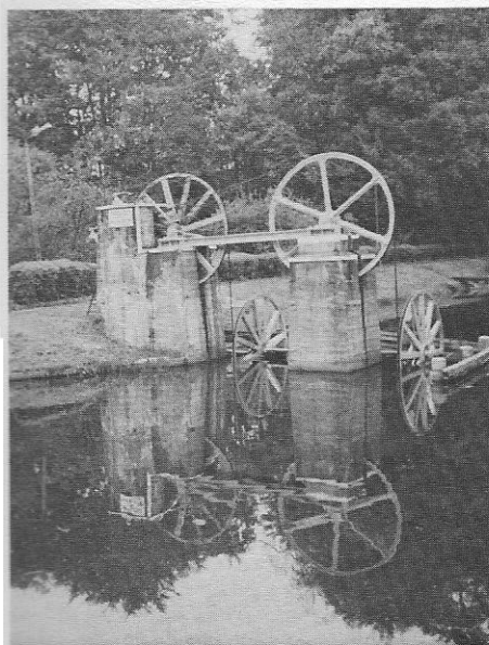
Pulley wheels and cables on the Buczyniec Incline, showing how the operating cables come from the side of the canal and turn at right angles in the water. The upper level of the canal is shown. (Squires photo.)
